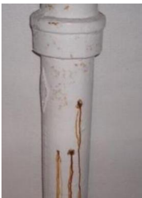
Drain pipe pinhole leaks. Pipes in wall leaking too??
