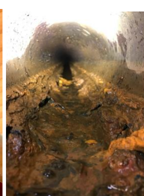
Inside drain pipe, note bottom pipe has thinned, likely area for pinholes
