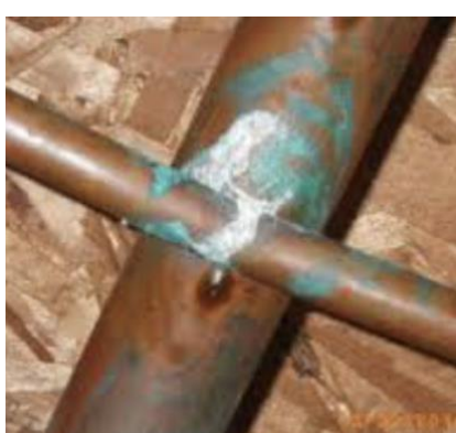
Leak where two pipes cross, have rubbed and created leakage
