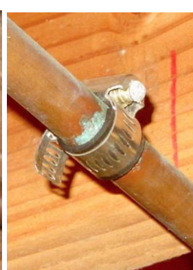
Temporary patch on water pipe, rubber under clamp
