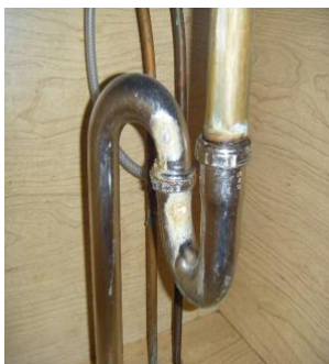
Sink drain trap corrosion caused by pinhole leakage
