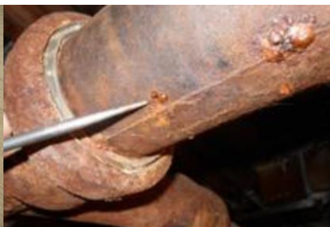
Pinhole leaks along bottom of drain pipe.
