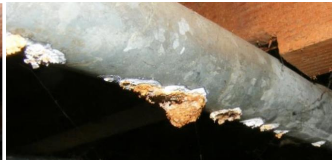
Advanced pinhole leakage with water dripping
