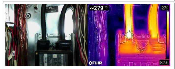
Above – The black cables were the main power feeds into the electric panel main breaker. Visually there was no apparent problem, however see IR photo to the right. Above – IR photo indicates one of the power entry cables into the main breaker is overheating, temperature of 279 Degrees F, which is a fire Hazard! Follow up, by an electrician, determined it was due to a loose lug connection at the main breaker.
