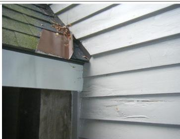
Kicker installed after damage was done to adjacent wall, note deterioration in siding. Kickers added after often are smaller than shown but just as effective.
