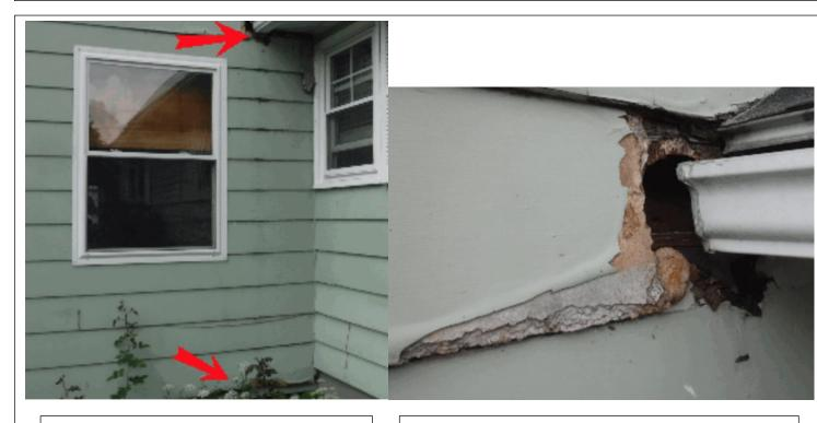
No kicker on upper roof, water has run down siding has stained it and deteriorated the siding. We often see window frames damaged too. With no kicker the water has rotted through the siding and likely has damaged the framing for the wall behind the siding.
