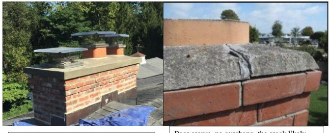
Large chimney with a custom-made crown. Note: Crown overhangs bricks. Chimney flues caulked to crown. Poor crown, no overhang, the crack likely due to no gap between crown and flue liner, thus when liner expanded with heat the crown cracked.
