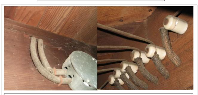
In some areas a heavier insulation was installed over the knob & tube wires as shown above. The heavier insulation had a shining material weaved in which is distinctive, helping the inspector not confuse this with a cloth insulation used over some insulation.
