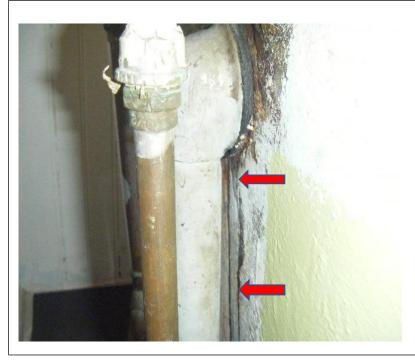
Above - red arrows show leakage from the tub overflow. The photo is of the tub overflow, often not visible during a home inspection.
